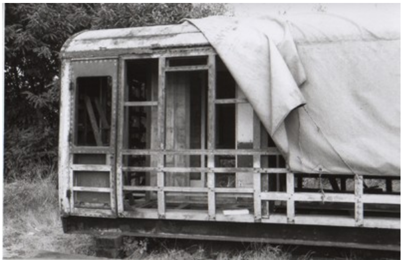
Body lowered onto new rail
