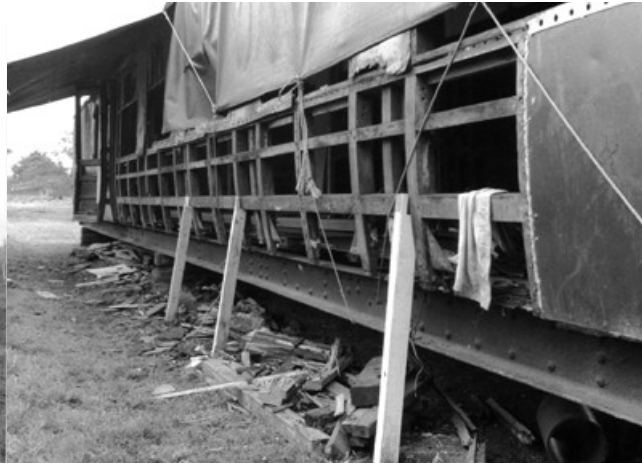
Rotten bottom rail removed.
