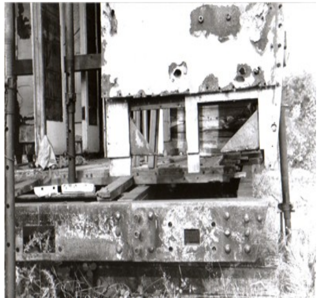
<Acrows in place
