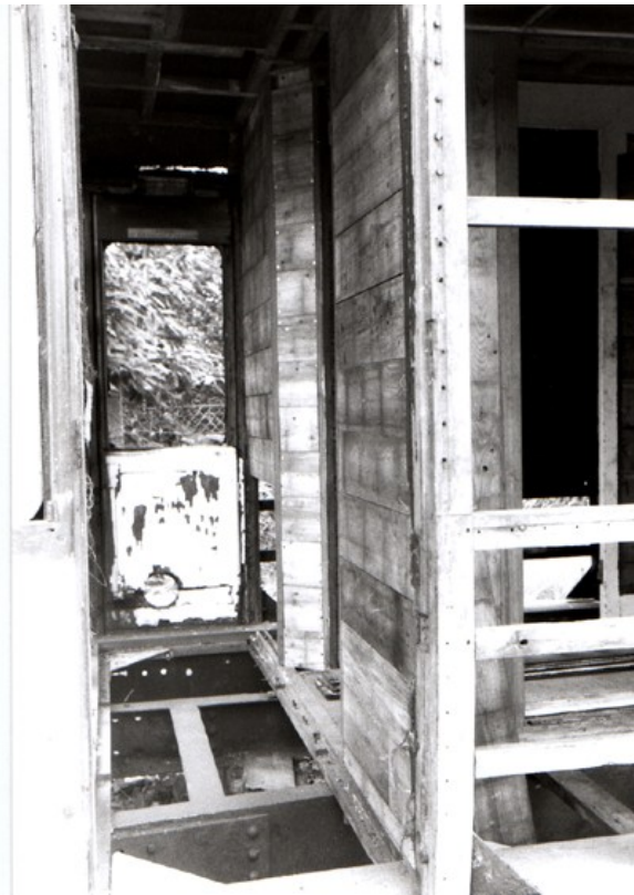
New toilet walls installed
