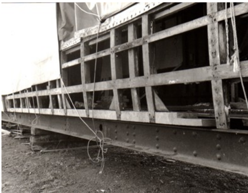
Section of new rail
