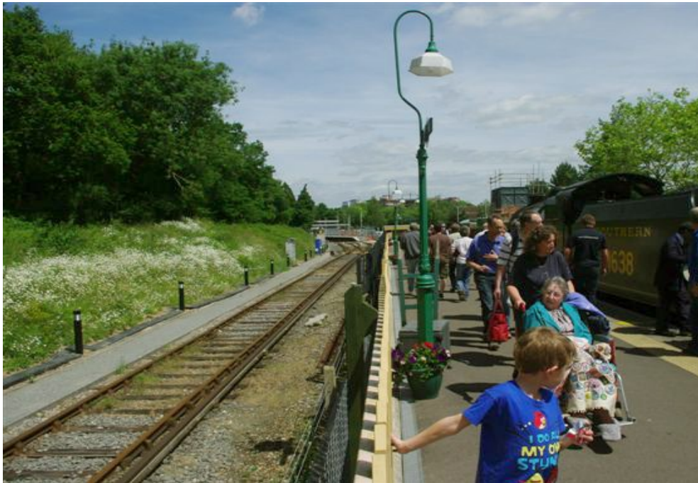
THE NEW EAST GRINSTEAD STATION WITH THE NATIONAL NETWORK LINE ON THE LEFT.
