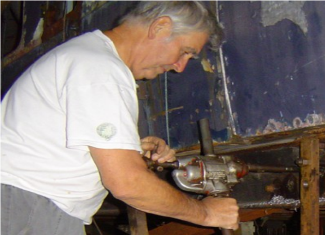
Drilling the truss rods
