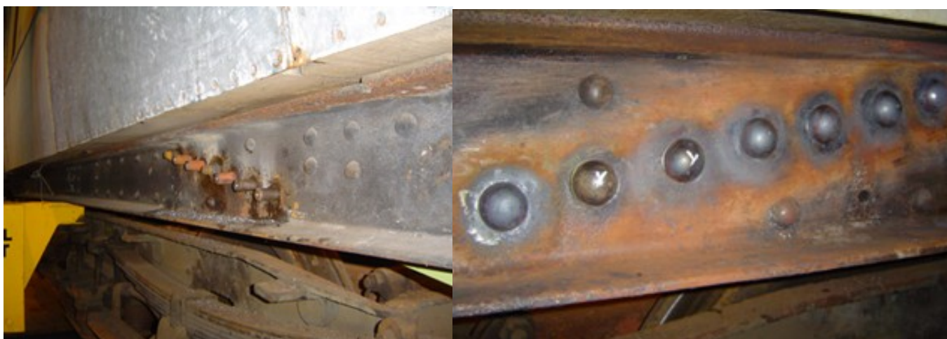
Rivets in place
