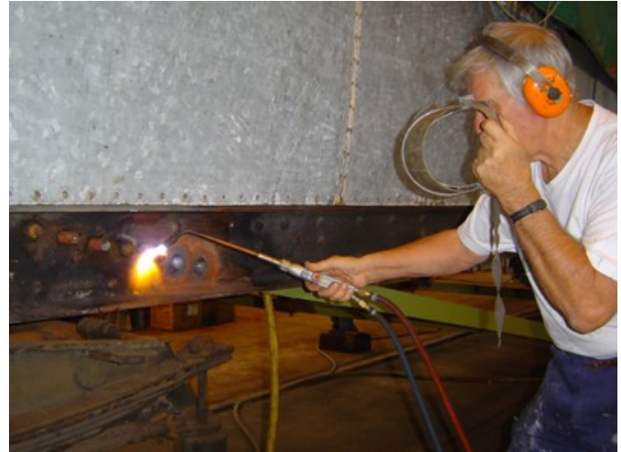
Heating up the rivets
