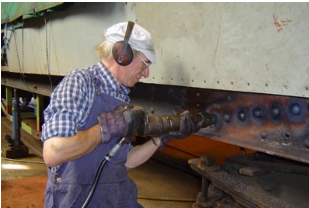
Hammering the rivets
