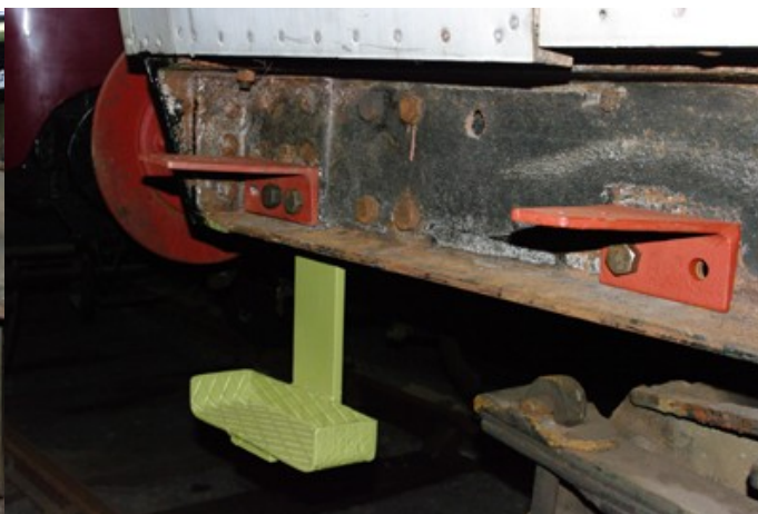
Above. New step and stepboard brackets.
